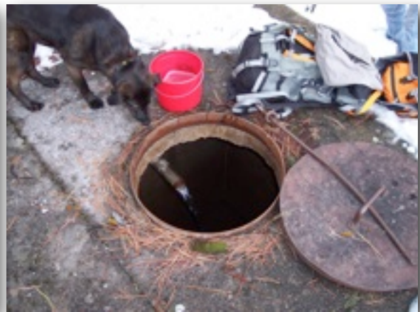
Figure 5. Pipe from Little Leroux Spring diversion to 200,000 gallon storage tank. This is the point where spring flow measurements are made
