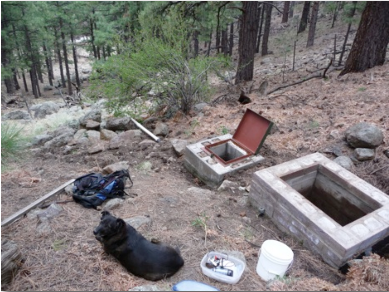
Figure 8. Big Leroux Spring box (at right), valve box just below, and drain outlet With PVC extension attached.
