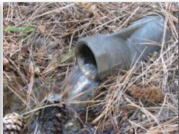
Figure 10. Big Leroux Spring drain outlet with four gallons per minutes flow.
