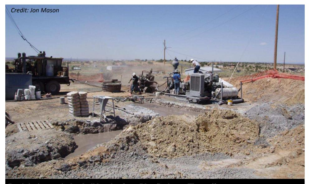
But it isn't practical to build a pipe from Blue Spring to Flagstaff. So well were drilled to intercept—short circuit—the water in the ground that otherwise eventually would have discharged at these springs.
