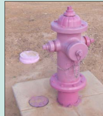
Reclaimed Water Fire Hydrant
